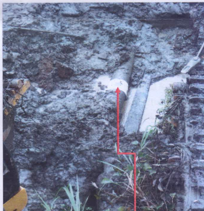
Fig C: Incident Facility after repair
