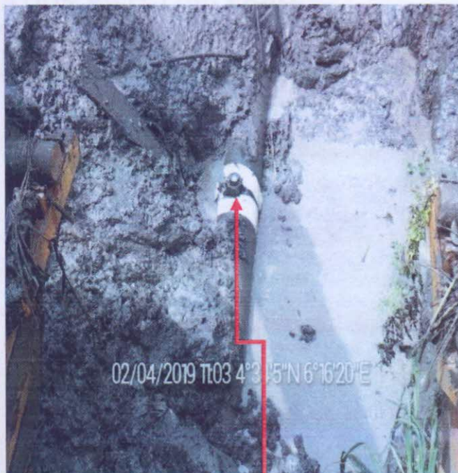
Fig B: The Incident Facility after excavation
